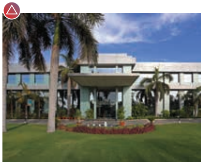
HEIL Changodar Plant
